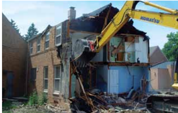
Demolition makes way for new buildings and parking lot.
